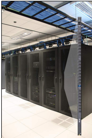
Figure 1: Switched PDUs enable organizations to define as many load segments as they require.
